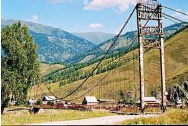
Bridge under Katun river near Tungur village
